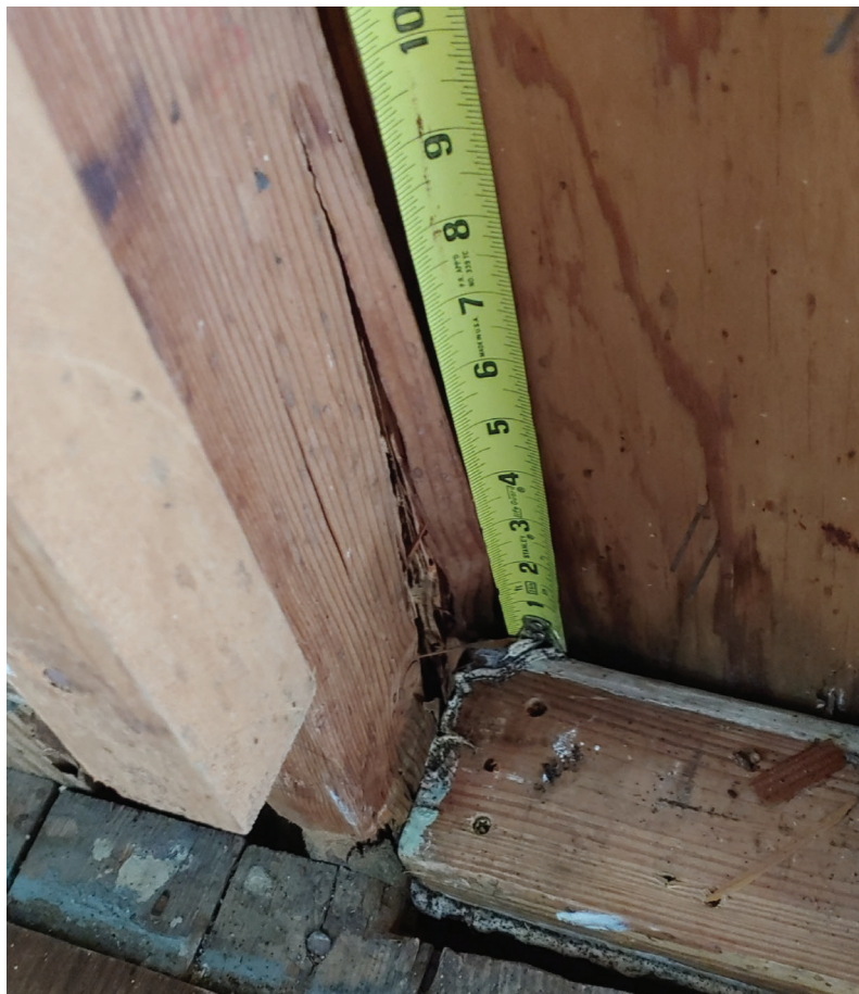
Figure 6 - Opening #1 - Rot at Bottom connection
