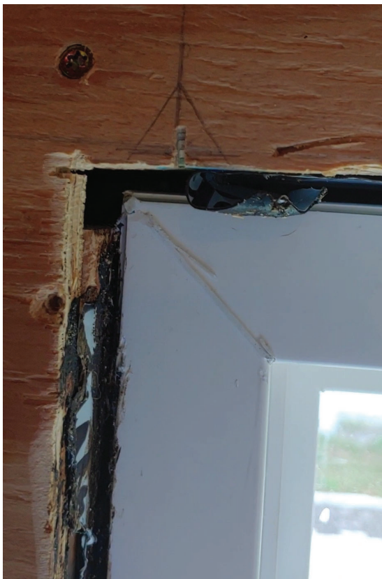
Figures 15 & 16 - Opening #3 - Structural is obstructed, Excessive Shim Gap
