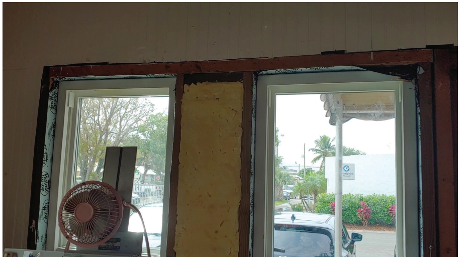
Figures 11 & 12 - Opening #2 - Header and Trimmer on Left Side are not properly installed.
