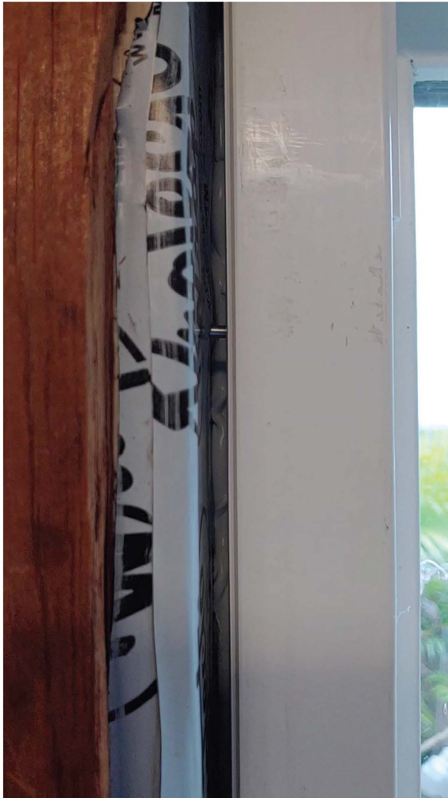
Figure 47 - Opening #16 - Excessive Gaps, Missing Shims
