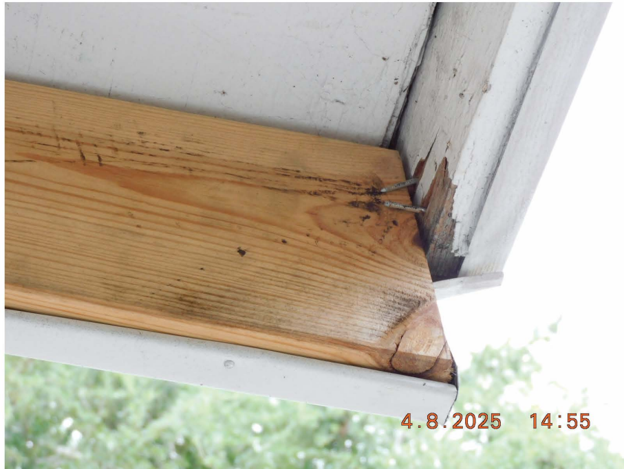
Figure 67 - Improper Fascia installation.
