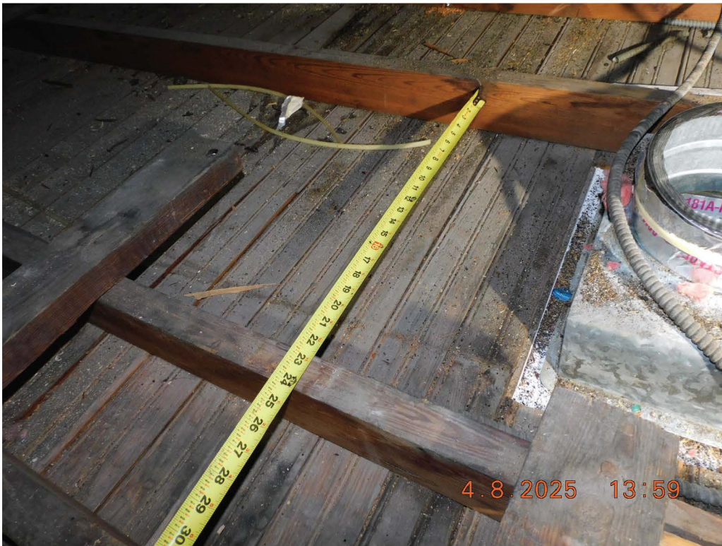
Figure 53 - Ceiling Joist Spacing in Original Section
