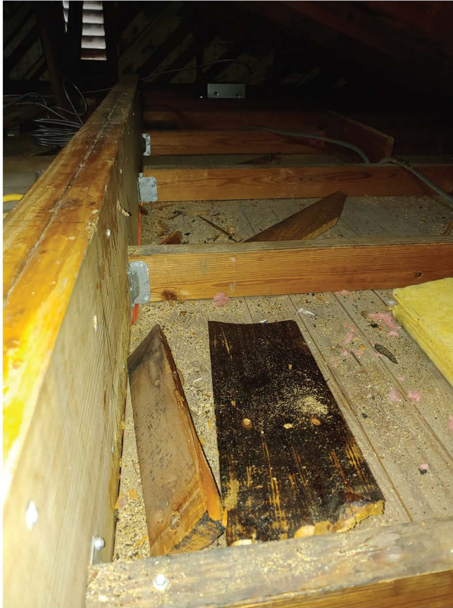
Figure 61 - Clip is missing screws in new section.
