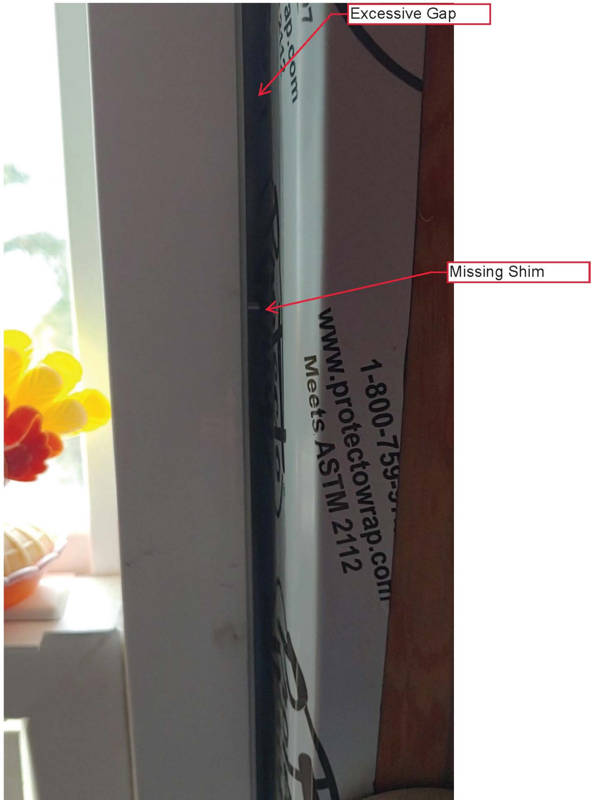
Figure 41 - Opening #8 - Excessive Gaps, Missing Shims
