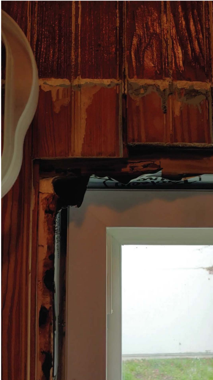
Figure 40 - Opening #7 - Wood Rot at Upper Left Hand Corner - Excessive Shim Spacing - Missing Shims
