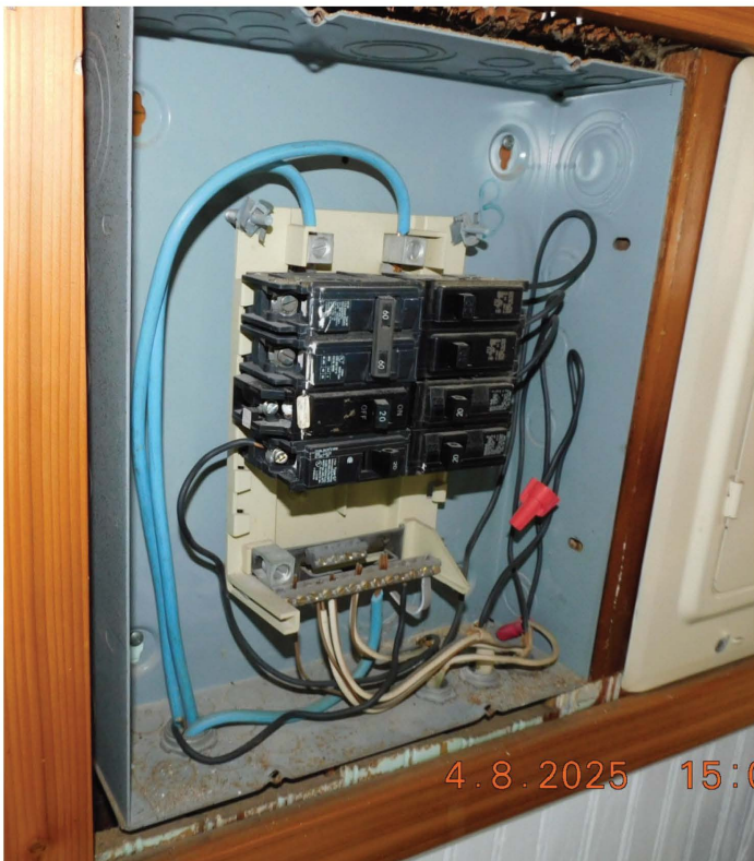
Figure 72 - Interior Electrical Panels A & B, Feeder Size Verification.
