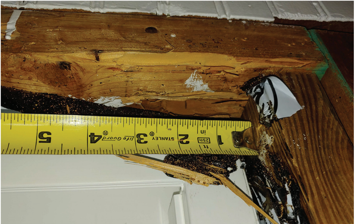
Figure 7 - Opening #1 - Rot at Top connection
