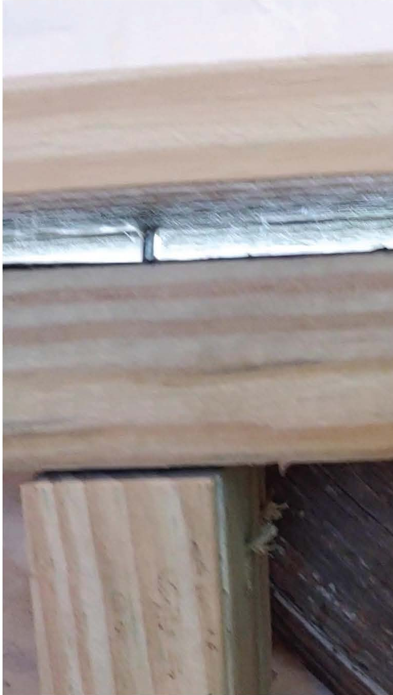
Figure 39 - Opening #7 - Excessive Gaps, Missing Shims
