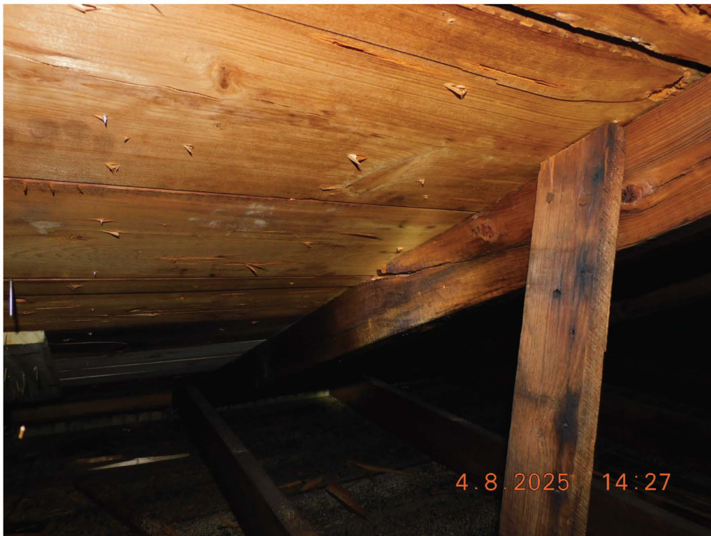
Figure 60 - Broken Rafter Needs to be Repaired
