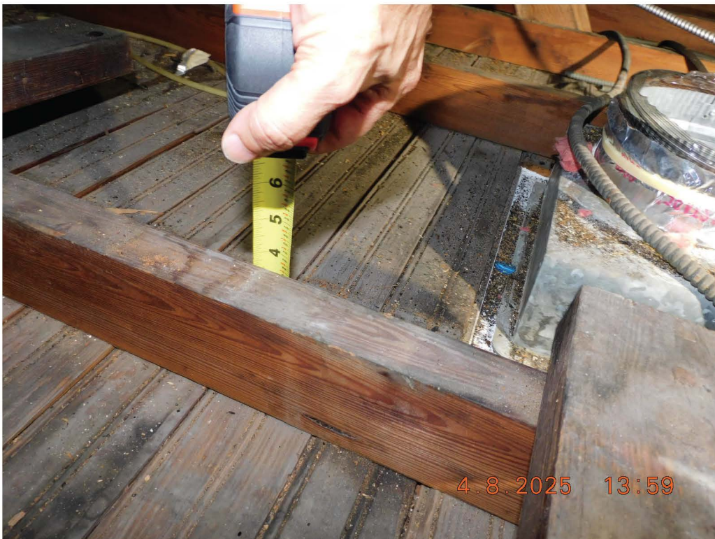
Figure 54 - Ceiling Joist Size in Original Section
