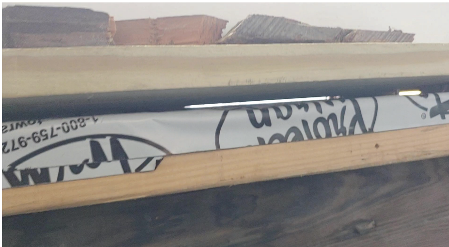
Figure 26 - Opening #5 - Improper Sill Installation Missing Shims Excessive Shim Gaps
