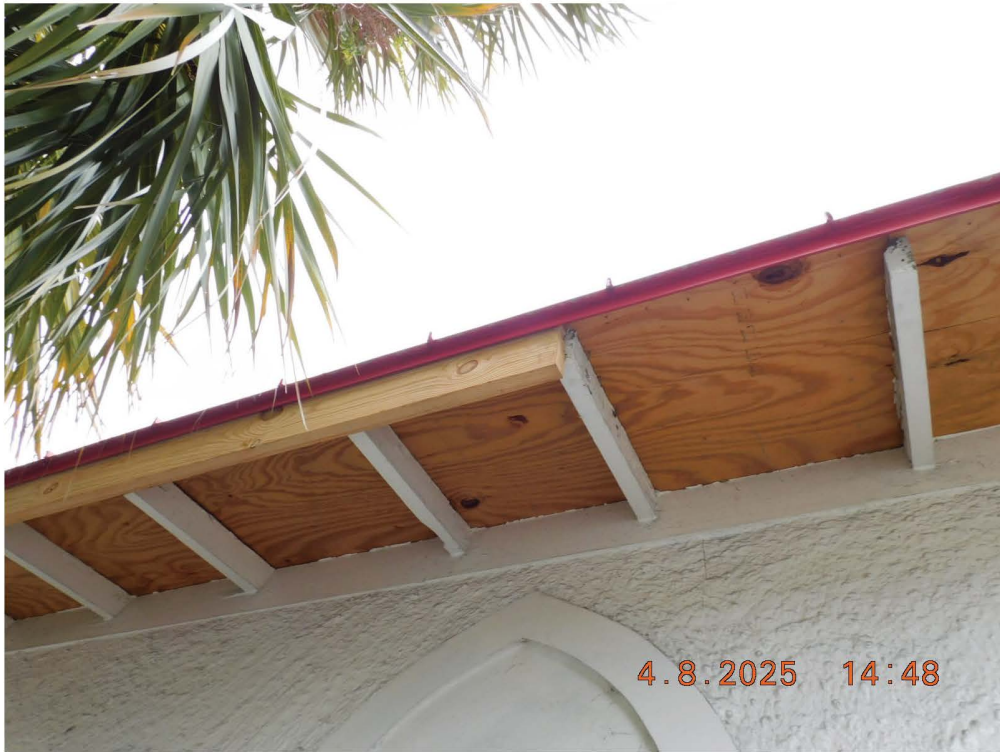
Figure 69 - Improper Fascia and Roofing Installation
