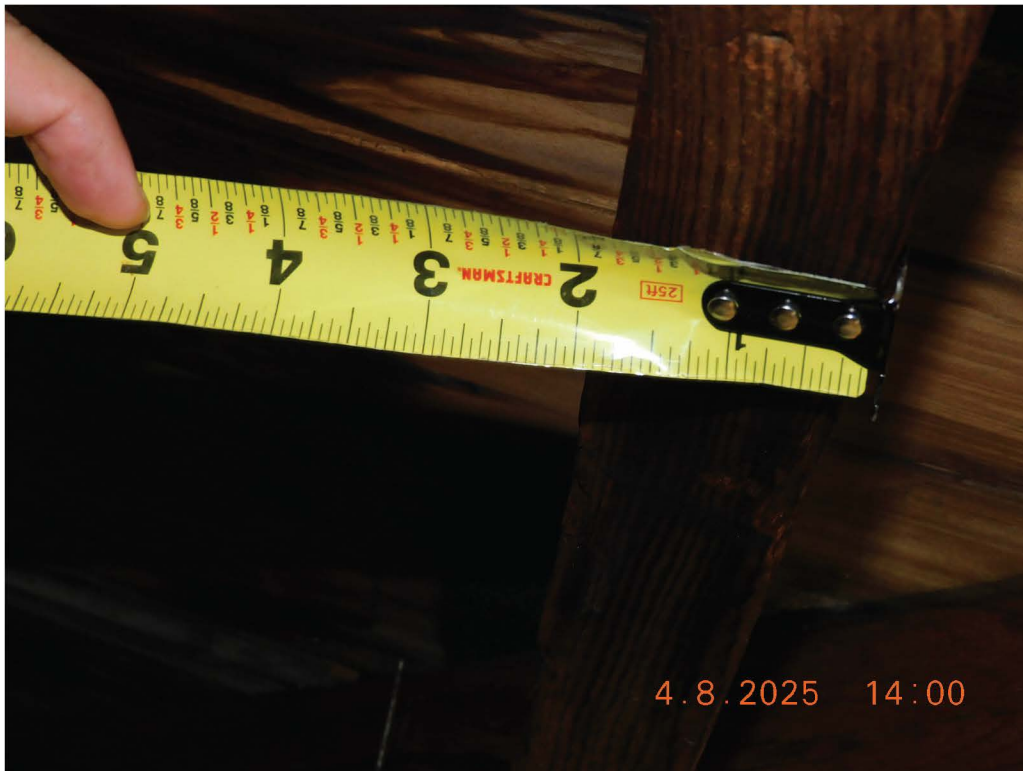
Figure 55 - Rafter Size in Original Section
