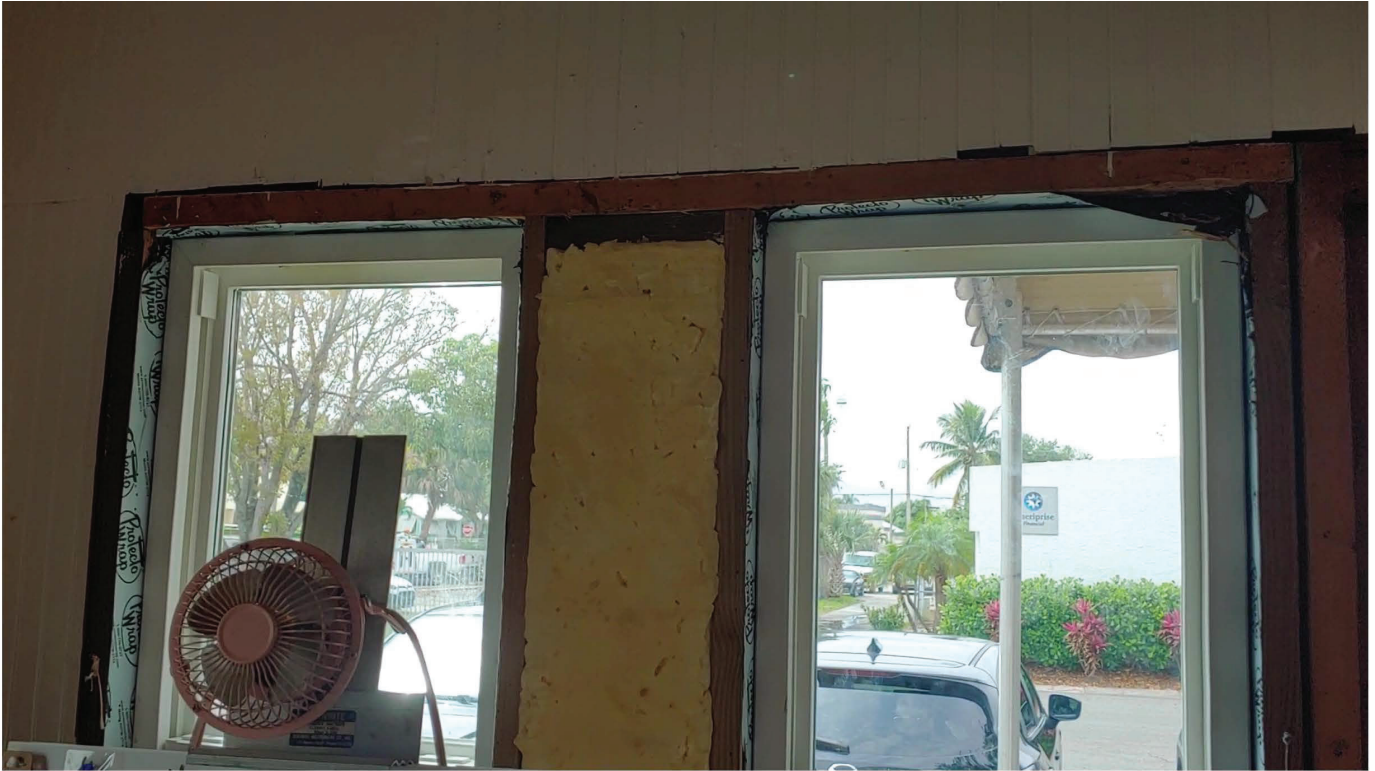
Figure 3 - Opening #1 - Improper Header
