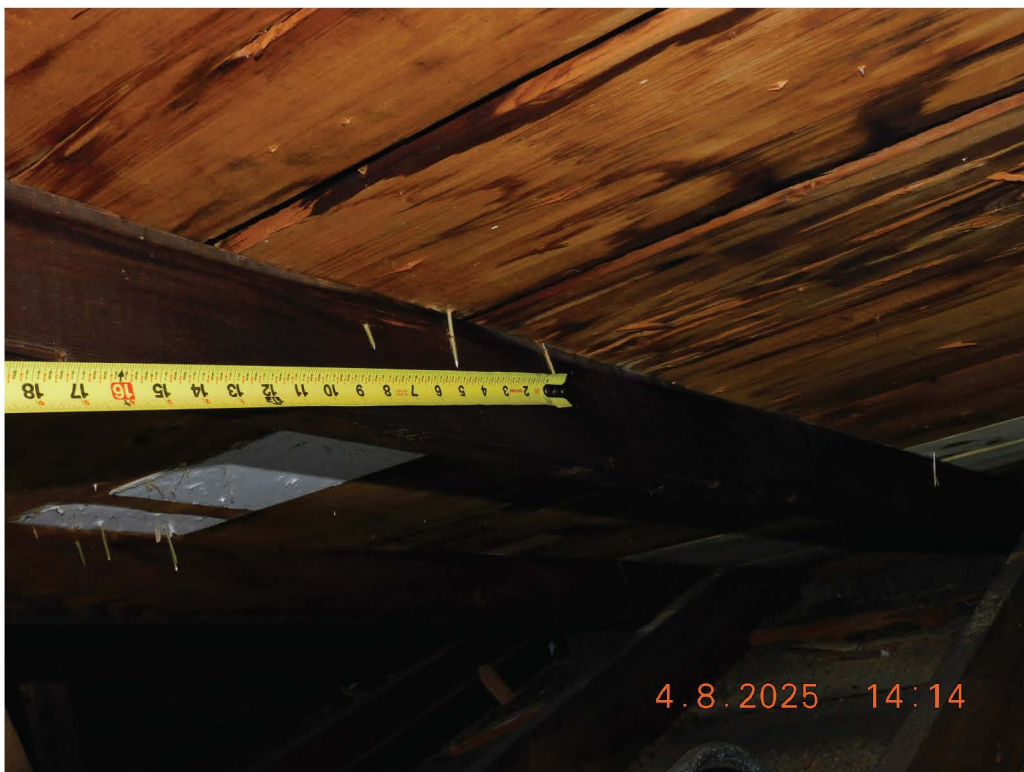
Figure 56 - Nails installed that missed the mark
