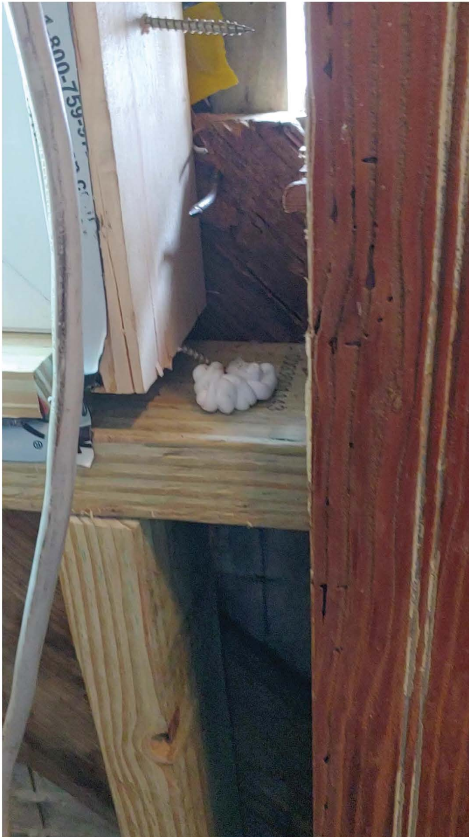
Figure 42 - Opening #8 - Improper Buck Installation
