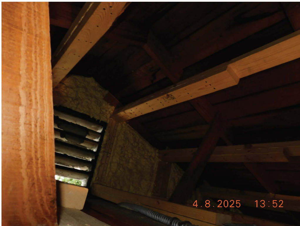
Figure 50 - Added Section at Front - Gable Reinforcement
