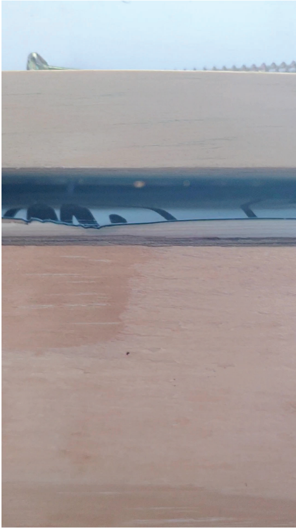
Figure 19 - Opening #3 - Missing shim, Insufficient sealant
