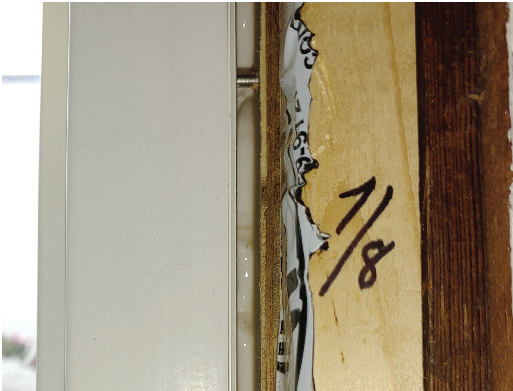
Figure 22 - Opening #4 - Double Buck with over sized Shim; missing shim Excessive shim gap
