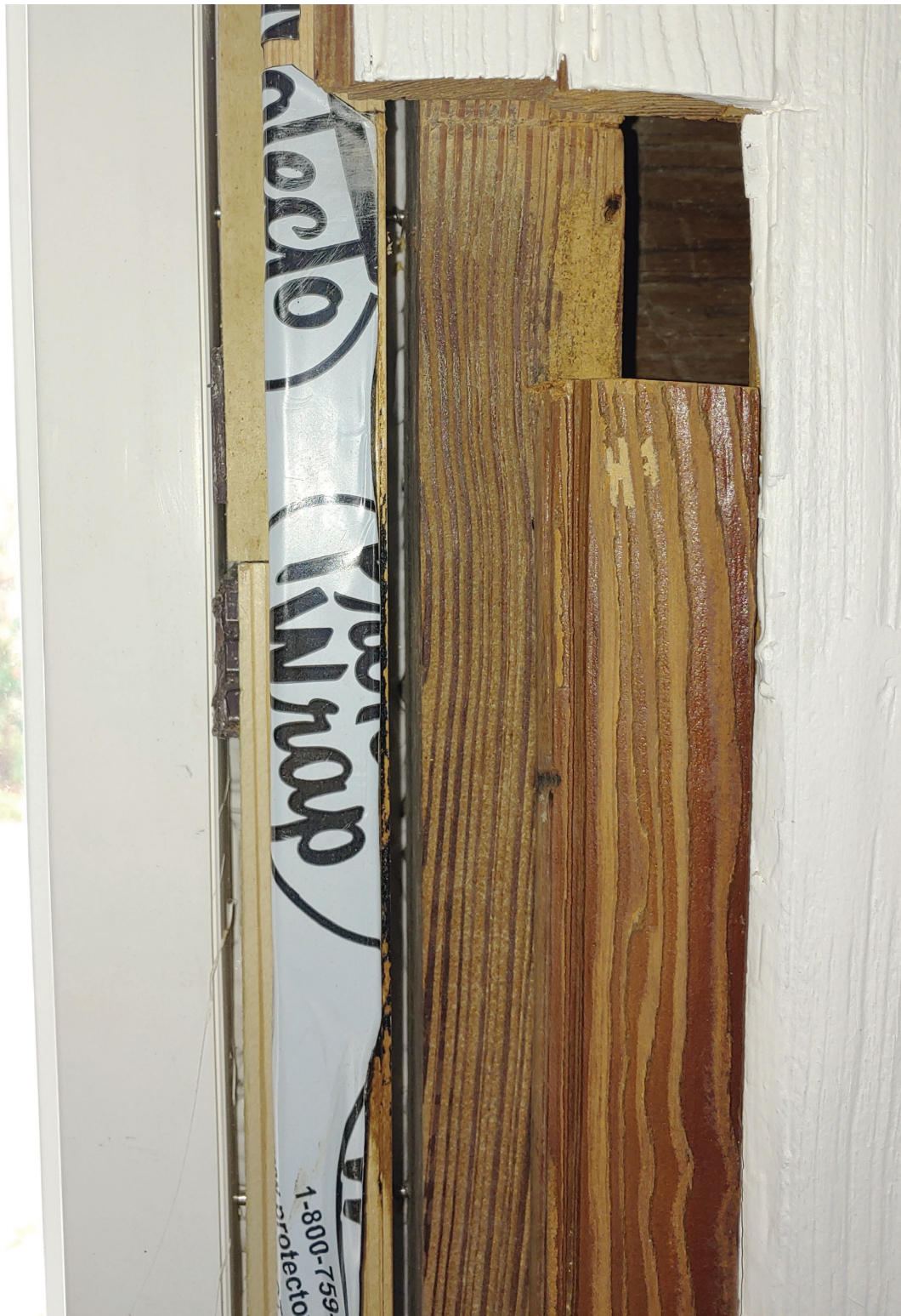
Figure 35 - Opening #6 - Improper Buck Installation Missing Shims & Excessive Space
