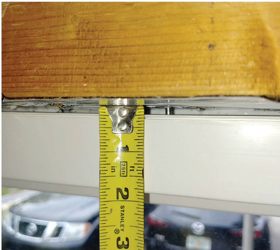
Figure 8 - Opening #1 - Shims are missing in several places, shim gap is excessive.
