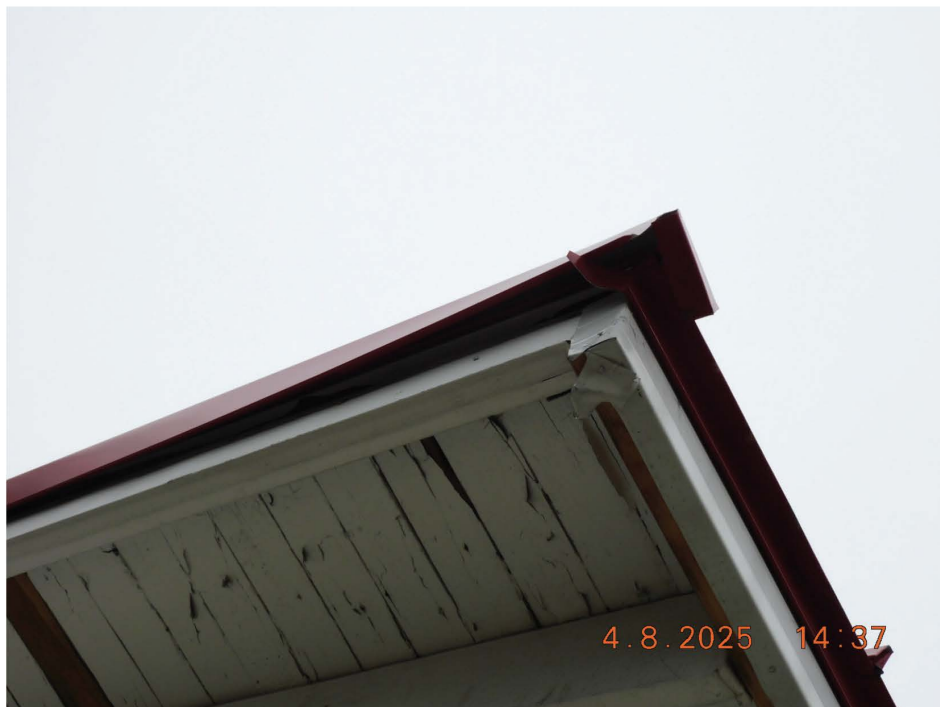
Figure 68 - Improper Fascia installation.
