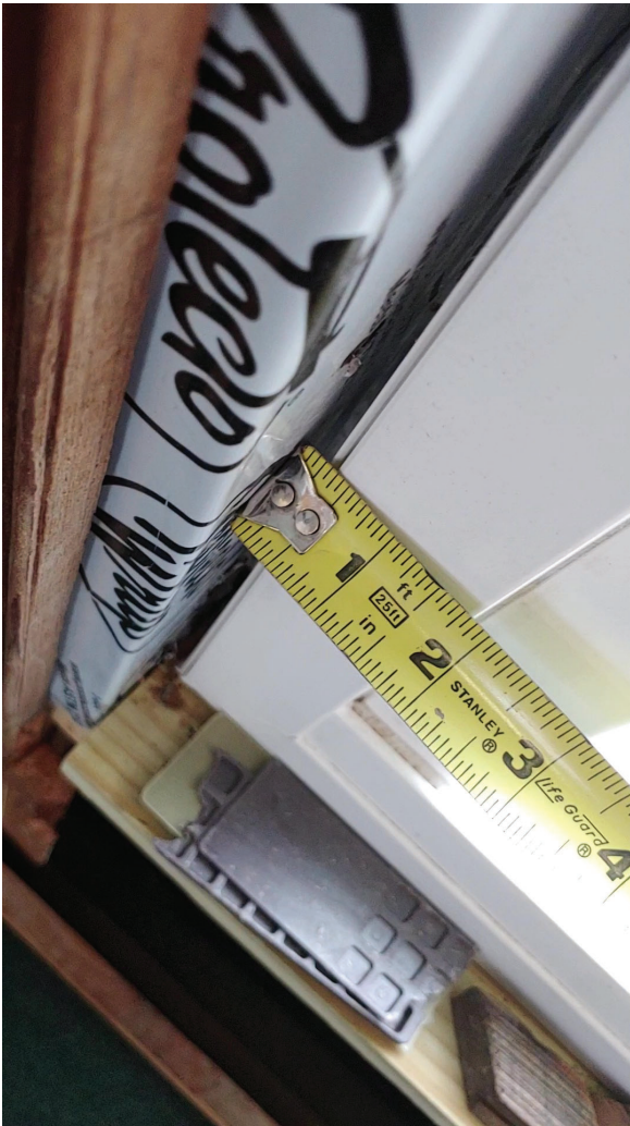
Figures 24 & 25 - Opening #5 - Oversized Shim; Missing Shim Excessive Shim Gaps
