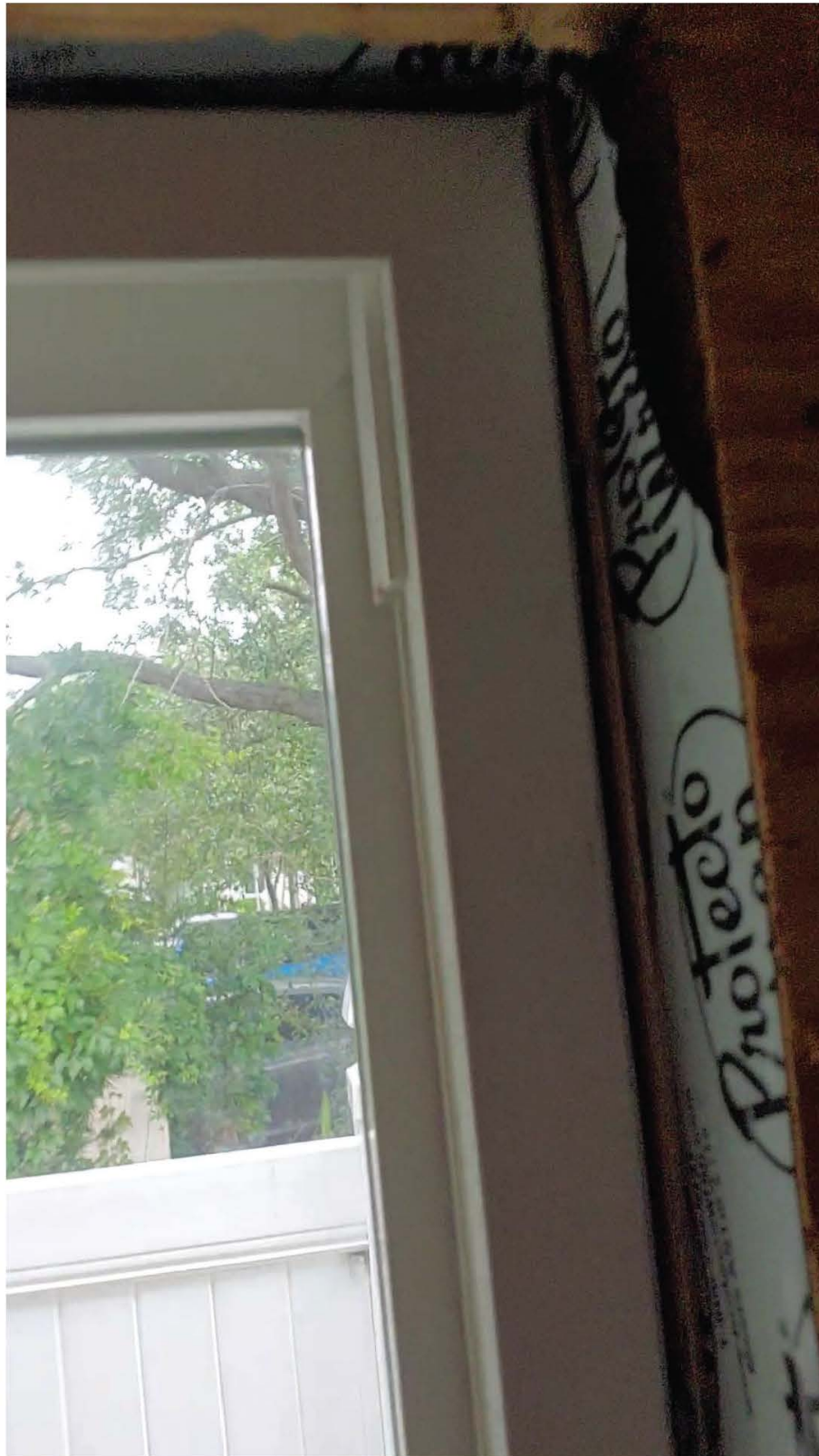
Figure 44 - Opening #10 - Excessive Gaps, Missing Shims
