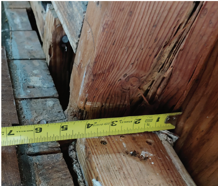
Figure 5 - Opening #1 - Rot at Bottom connection
