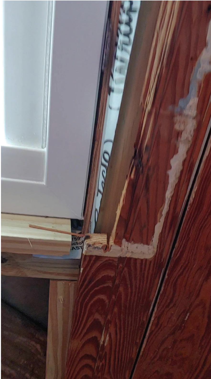
Figure 37 - Opening #7 - Improper Trimmer/Buck Installation Excessive Space
