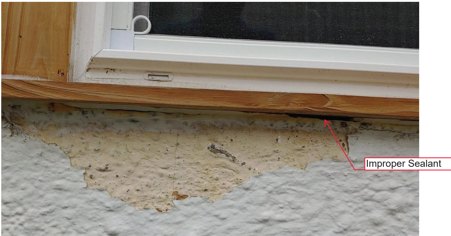
Figure 29 - Opening #5 - Improper Sill Installation; Improper sealant application.
