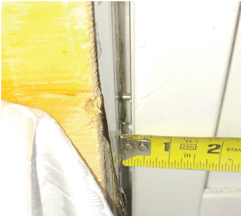
Figure 18 - Opening #3 - Missing shim Excessive shim gap
