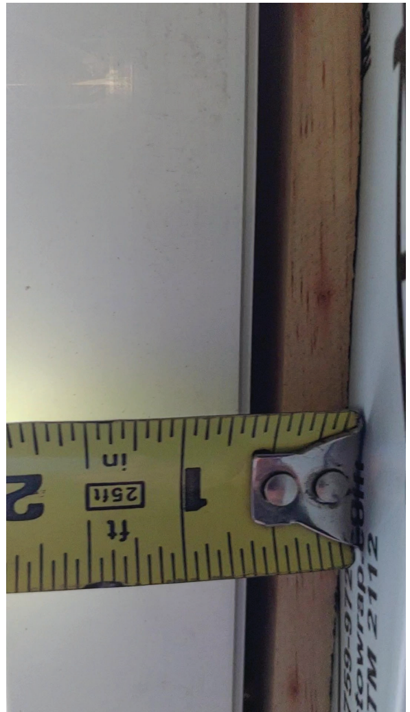
Figures 24 & 25 - Opening #5 - Oversized Shim; Missing Shim Excessive Shim Gaps
