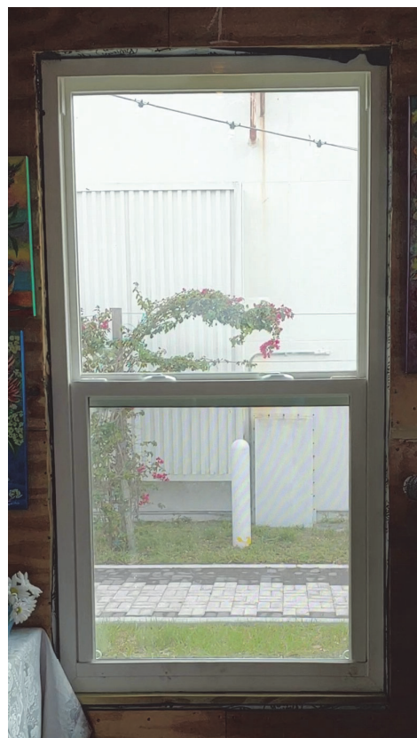
Figures 15 & 16 - Opening #3 - Structural is obstructed, Excessive Shim Gap
