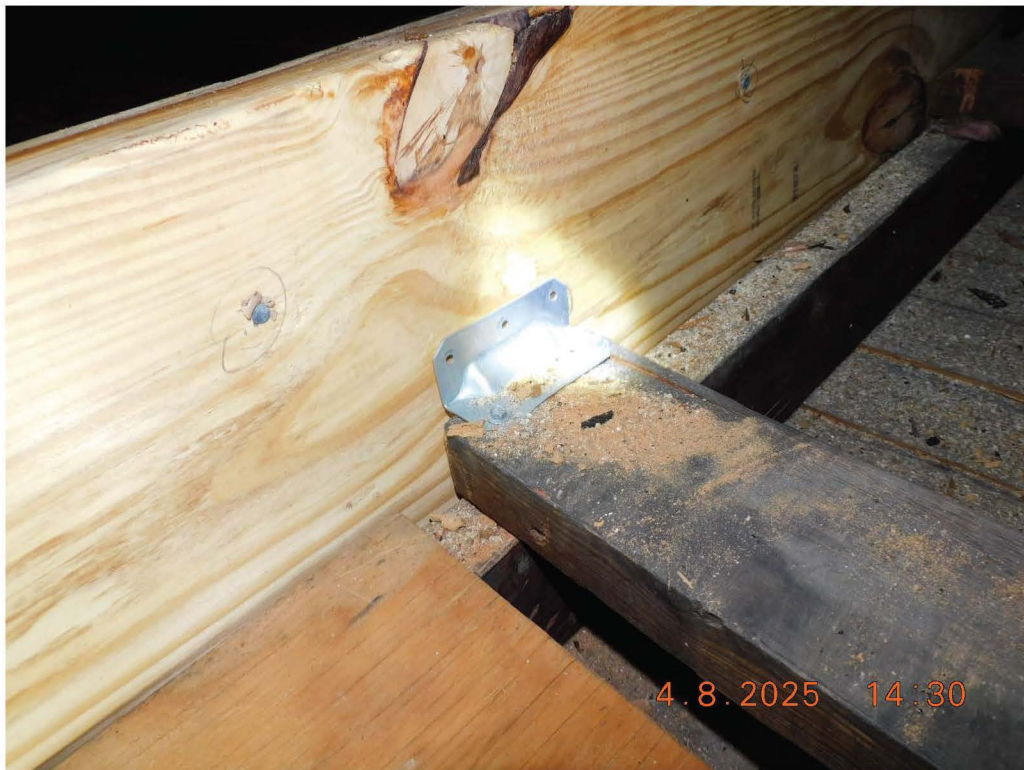
Figure 62 - Clip is missing screws in new section.
