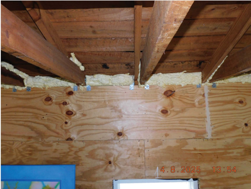
Figure 51 - Added Section at Front - Clipped Ceiling Joists
