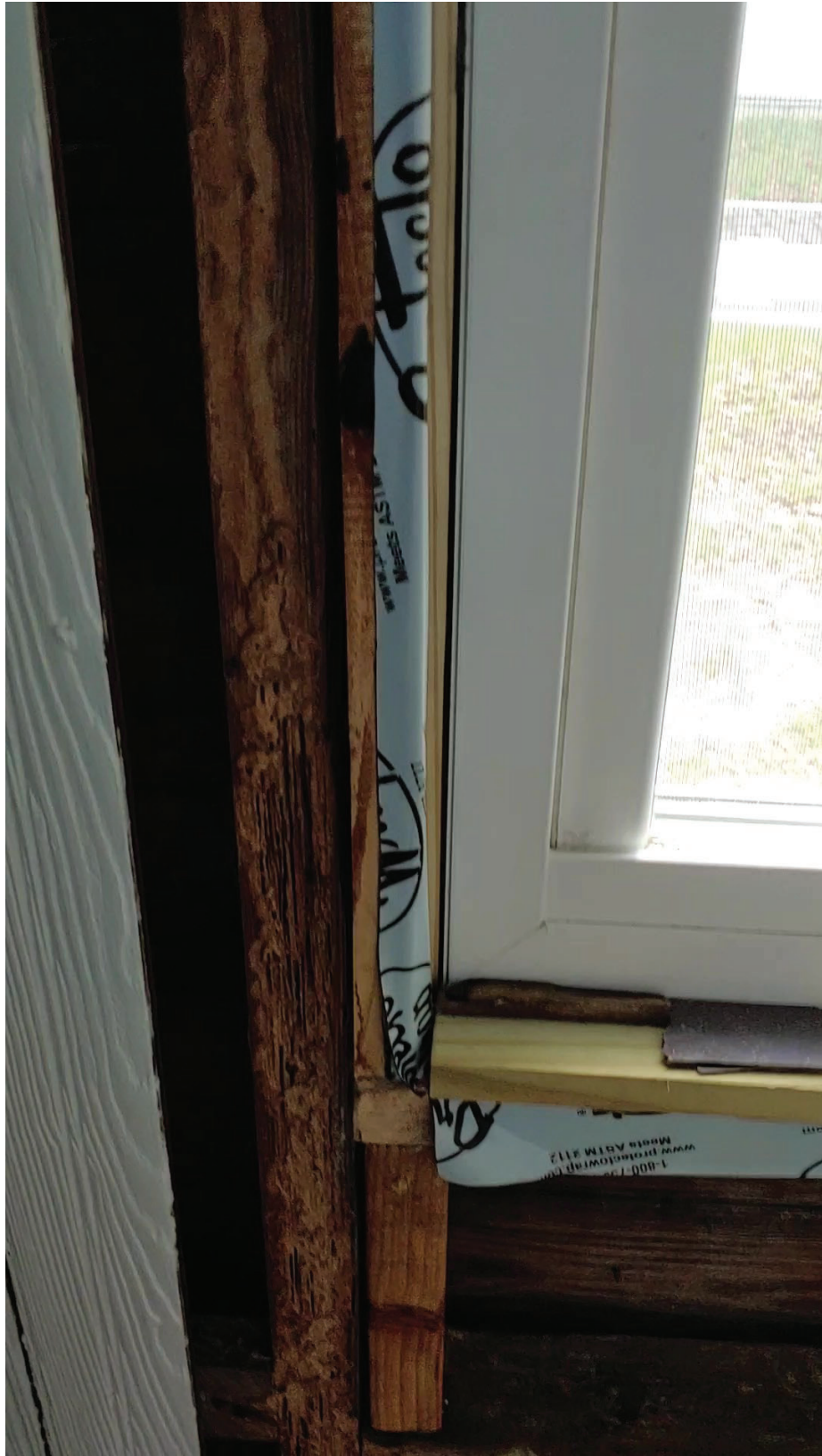
Figure 34 - Opening #6 - Improper Buck Installation; Trimmer Rot? Buck or Sister?
