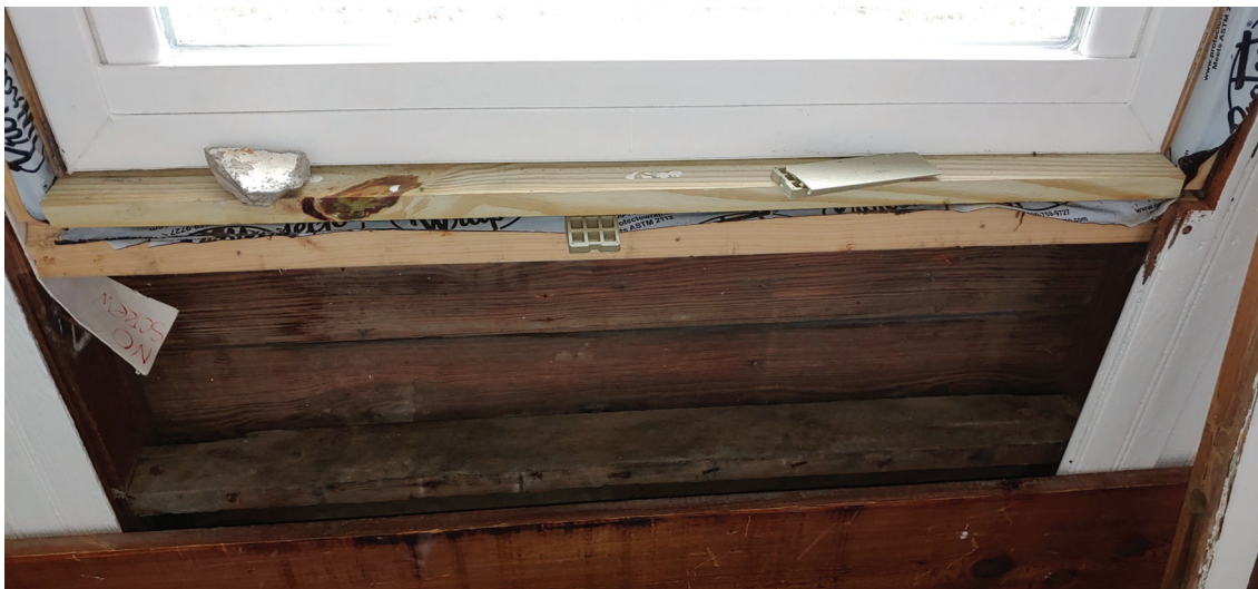
Figure 23 - Opening #4 - Missing Jack Studs to support Sill; No Functioning Trimmer Studs
