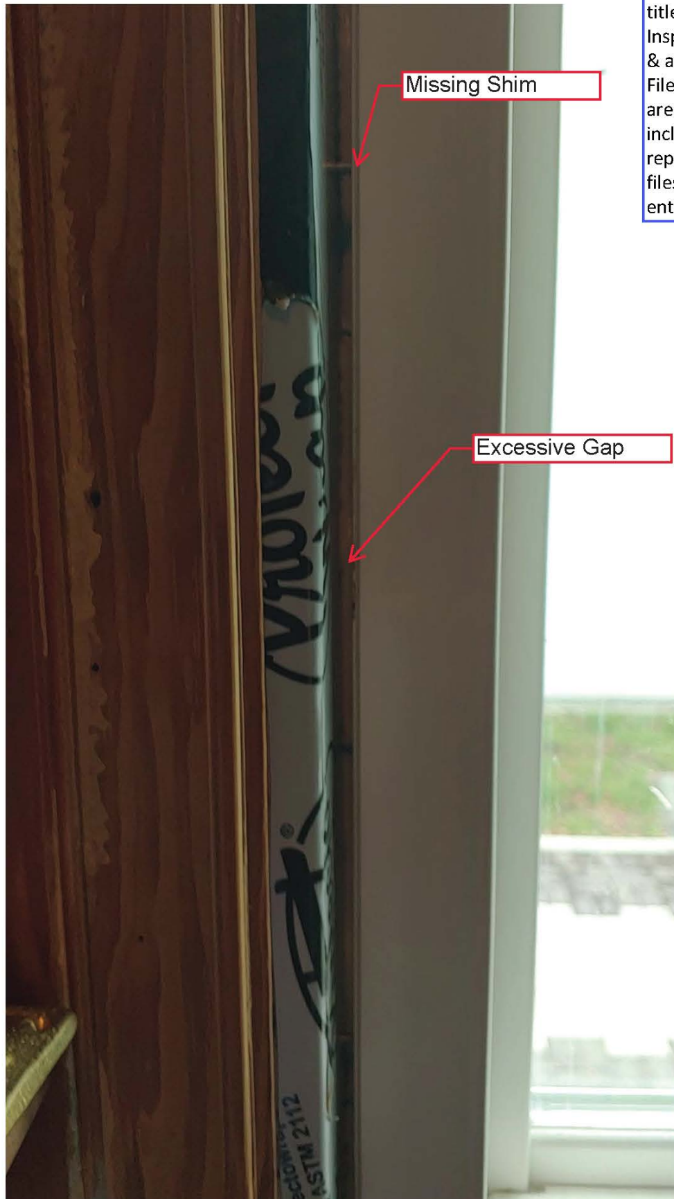
Figure 38 - Opening #7 - Excessive Gaps, Missing Shims
