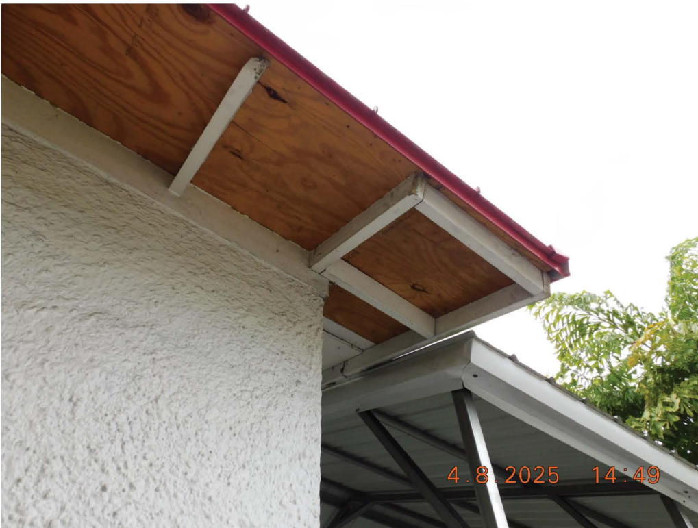
Figure 70- Improper Fascia and Roofing Installation
