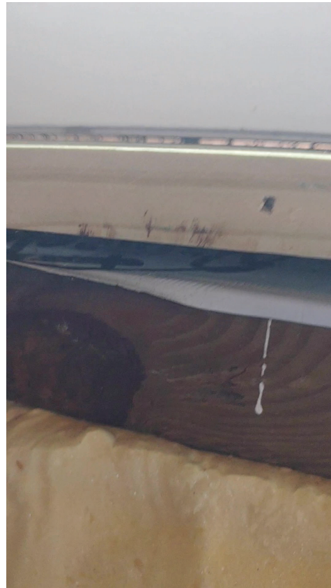
Figures 13 & 14 - Opening #2 - Sill not Installed, shimmed or sealed properly
