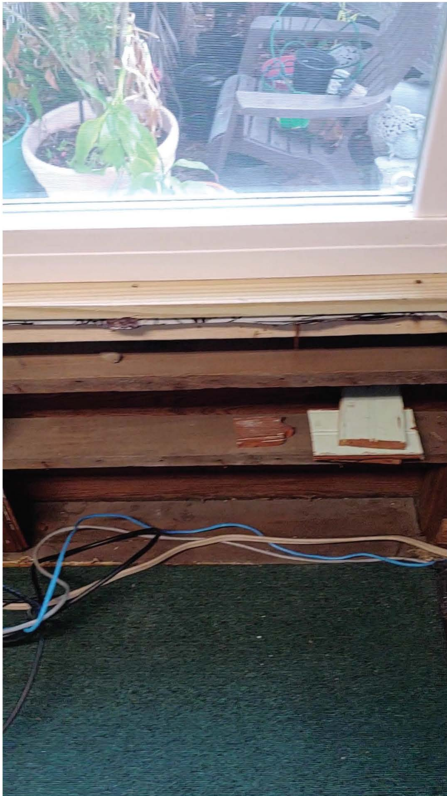
Figure 48 - Opening #17 - Improper Sill Installation - Missing Jack Studs
