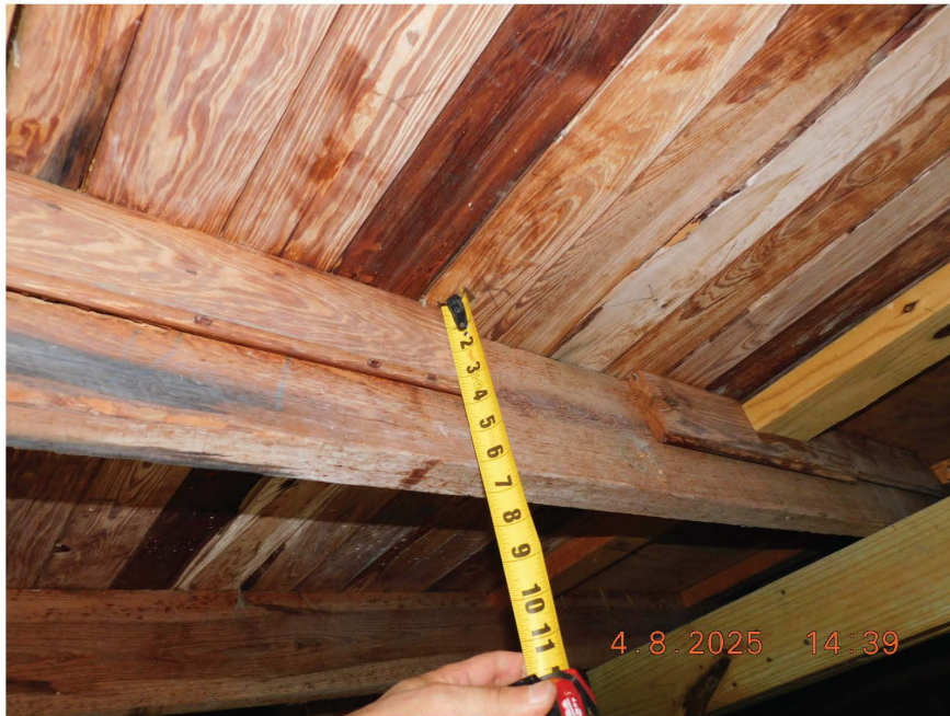
Figure 64 - Floor Joist Measurement
