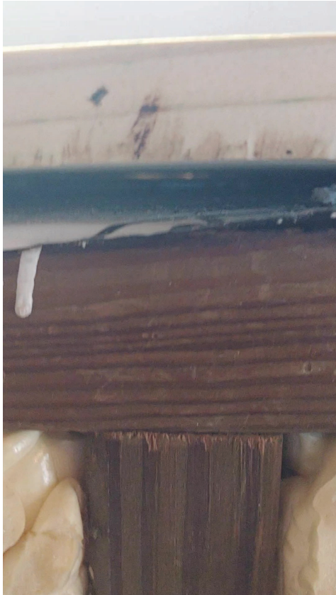
Figures 13 & 14 - Opening #2 - Sill not Installed, shimmed or sealed properly
